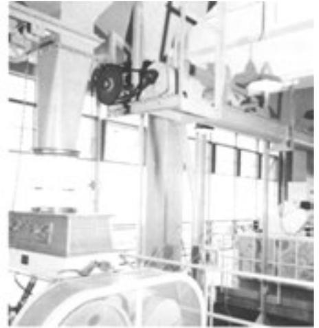
*Top Right* - Over 40 feet of screw conveyors carry malt and rice from storage to mills in this factory.
