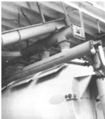
*Center Left* - Typical installation provides close fitting gates and connections,
