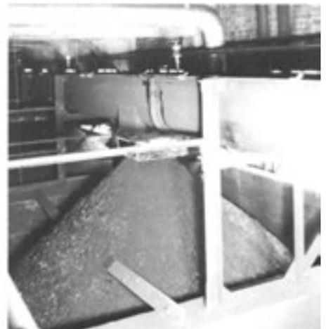
*Center Right* - Helicoid screw conveyor delivers 50 tons of coal per hour to boiler room bunkers.
